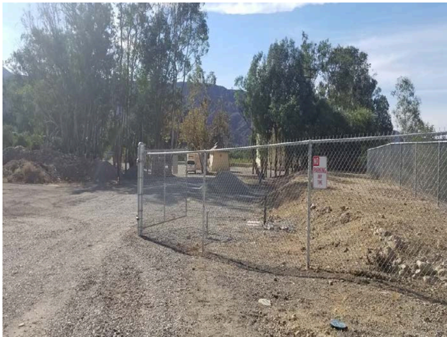
Photograph 2. View of existing wells, tanks, and pumps infrastructure within BSA, east of San Antonio Creek, facing south (Unit A). Note eucalyptus trees within BSA. November 13, 2018.
