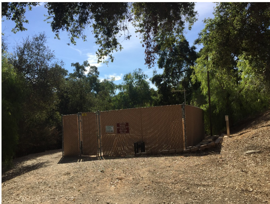
Photograph 4. View of existing Fairview Pump station within BSA, facing south (Unit B). November 13, 2018.
