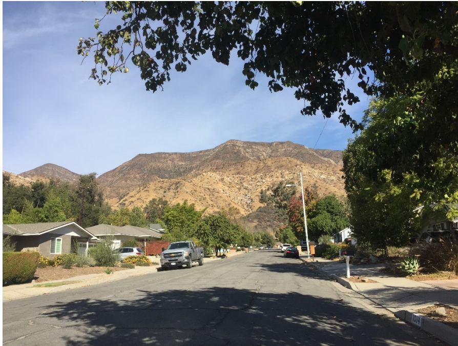
Photograph 5. View North Sunset Place of existing pipeline alignment within BSA, facing north (Unit B). Note ornamental vegetation surrounding the project footprint. November 13, 2018.
